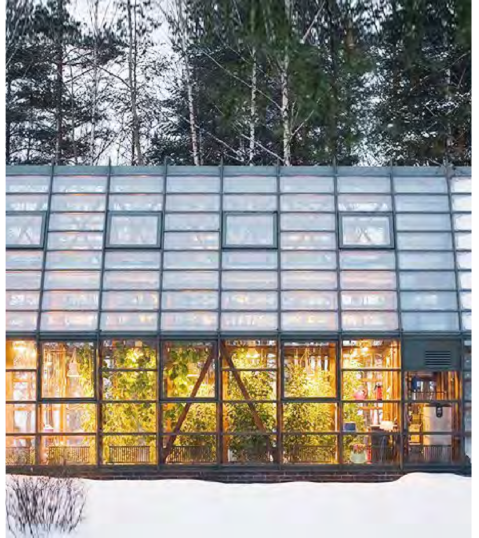
PIROGOVO GREENHOUSE - TOTAN KUZEMBAEZ ARCHITECTS
