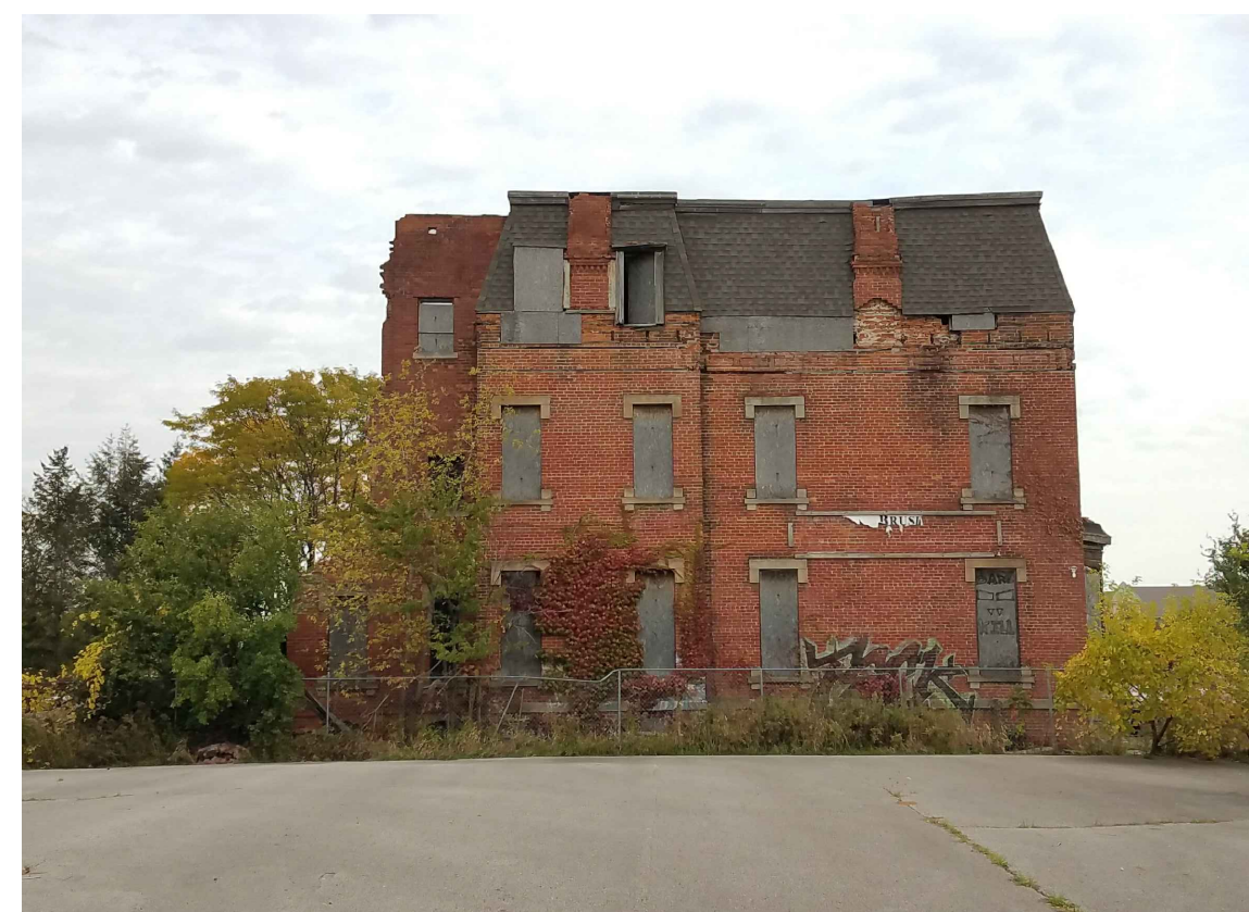
8 WEST ELEVATION PHOTO
