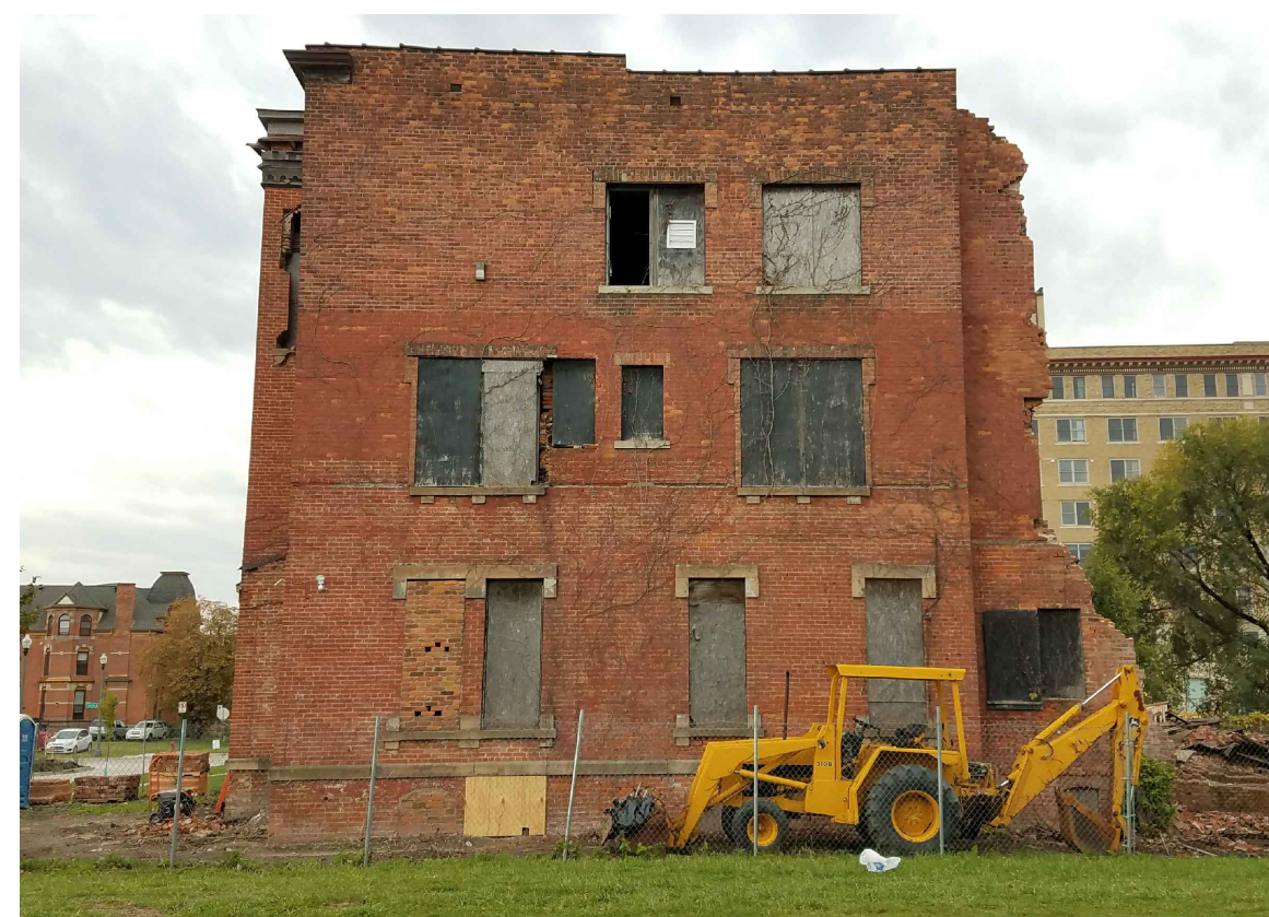
6 EAST ELEVATION PHOTO
