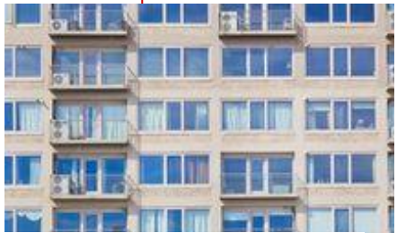
REGULAR WINDOW PATTERN (CARLTON LOFTS)
