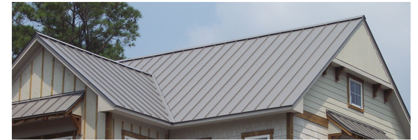
STANDING SEAM METAL ROOF
